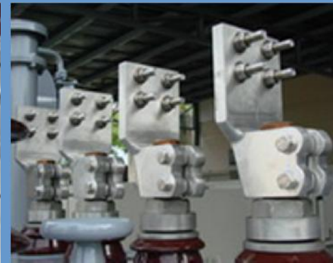
LV terminal connector (pad type)
