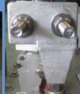
HV terminal connector
