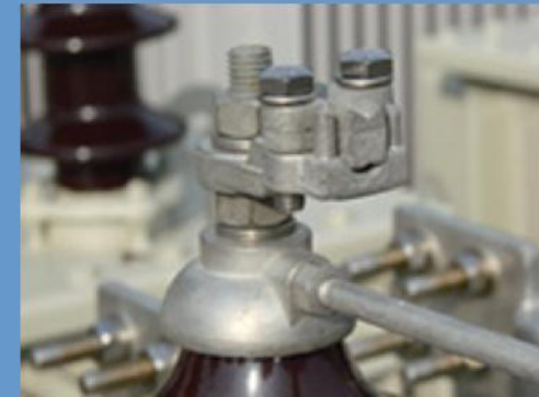
HV terminal connector
